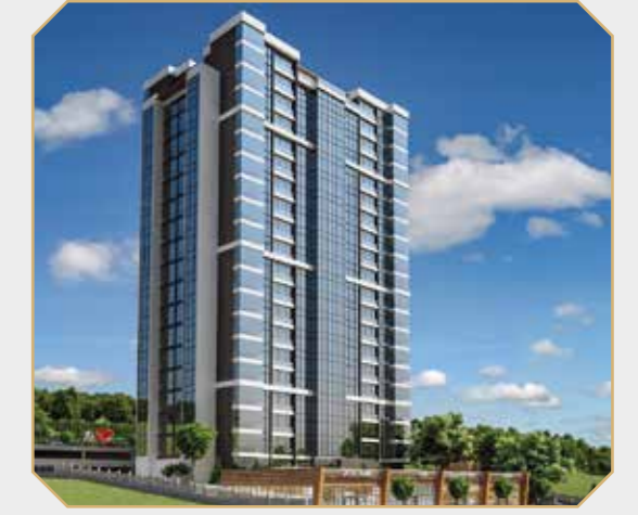
BP TOWER WESTAR
